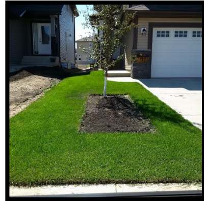
Area around tree is unfinished
